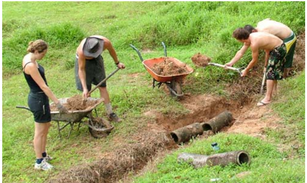
Students working on drainage for a soccer field.
