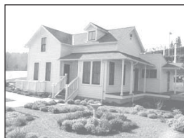
Restored Chase House
